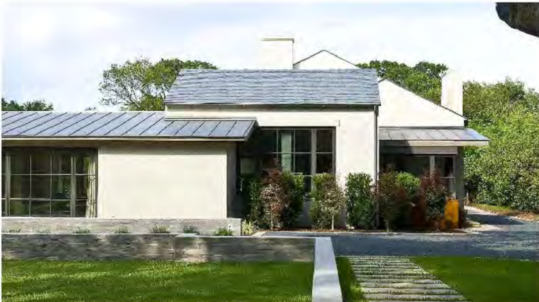
14 THIS HOME COMBINES PAINT GRIP AND SLATE ON ITS ROOF
