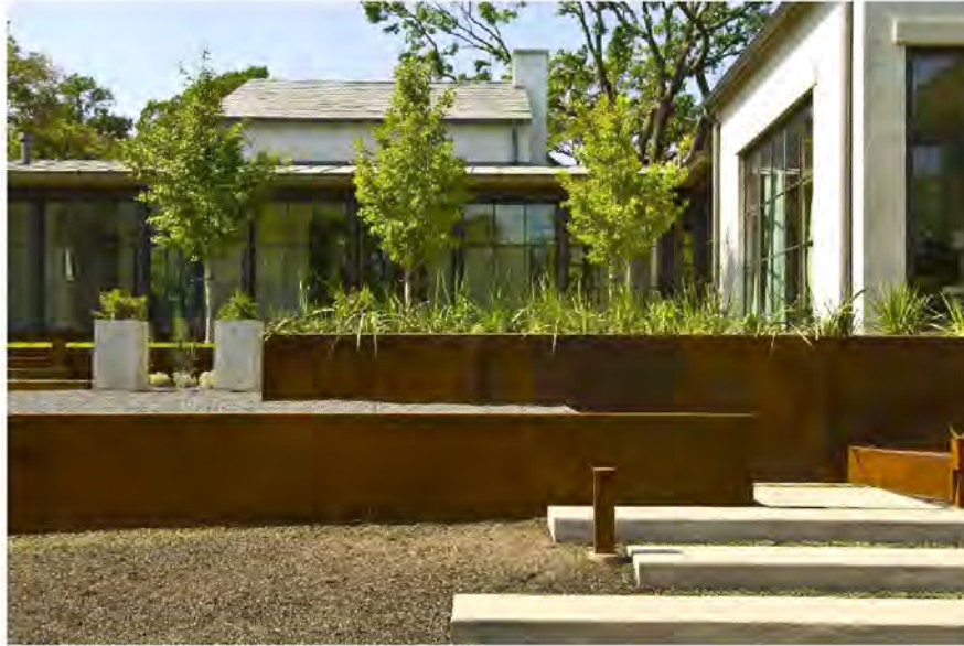
19 AN EXAMPLE OF COR-TEN RETAINING WALLS WITHIN A COURTYARD
