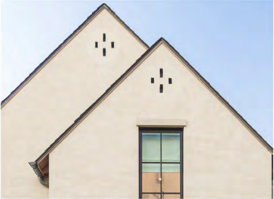
12 AN EXAMPLE OF PORTLAND CEMENT STUCCO
